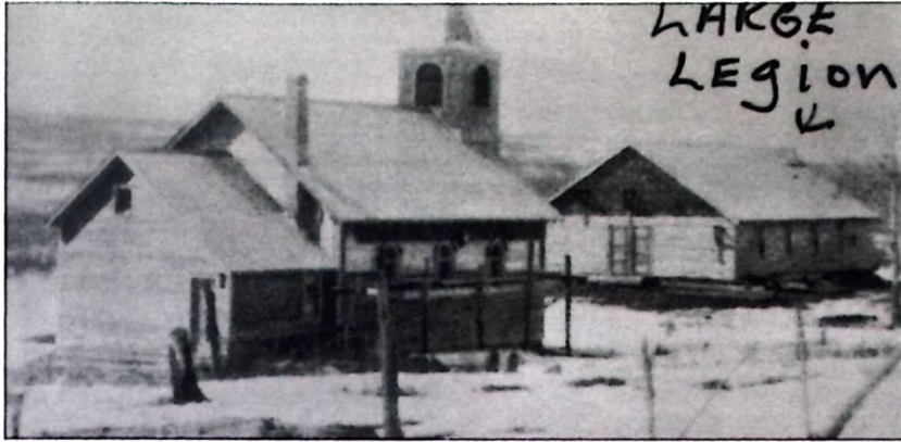
The Large Legion identified in the picture is the building that was purchased for $5.00 from the St. Paul School District. The original Legion not shown in picture was located to the left (south) of the church.
