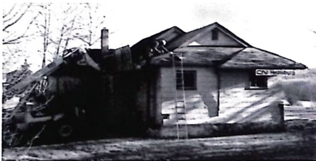
CNR Station Roof Restoration
